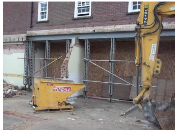
Rear Elevation January 2012
