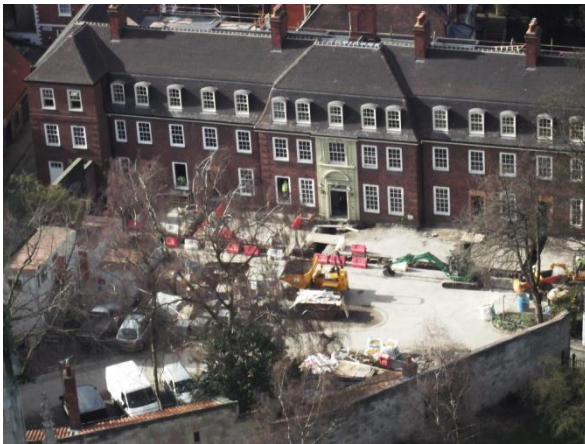
Utilities trenches being dug – March 2012
