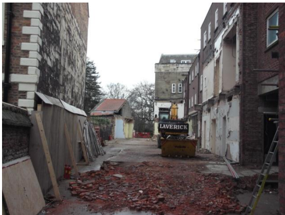
Rear Elevation January 2012
