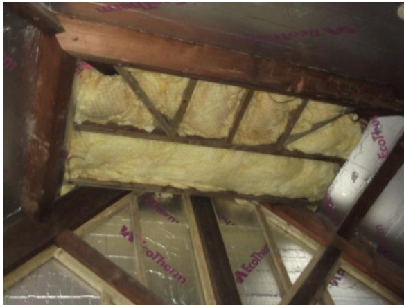
The Clifford Apartment– Roof Timbers/Insulation
